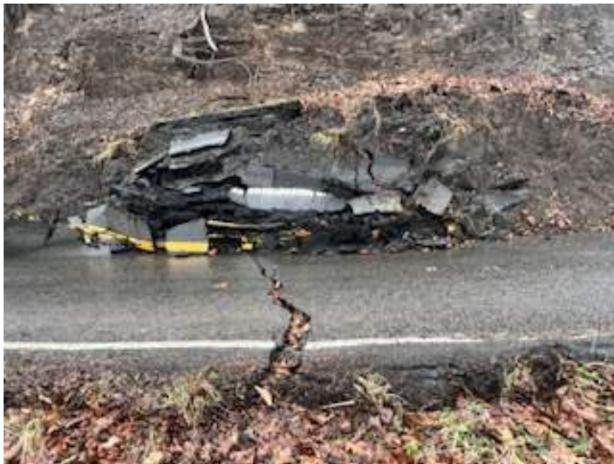
Figure 647: Damage from Landslide Event on Route 91
